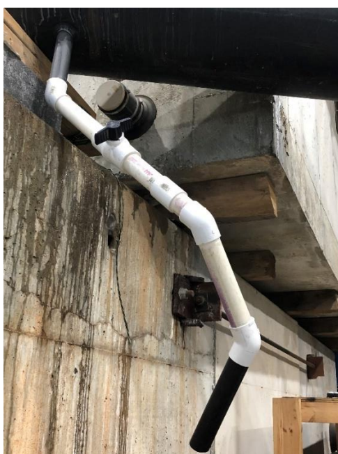
Figure 8 Photograph of Background Sampling Port
