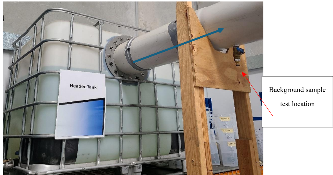
Figure 5 Photo of the Installed Constant Head Tank
