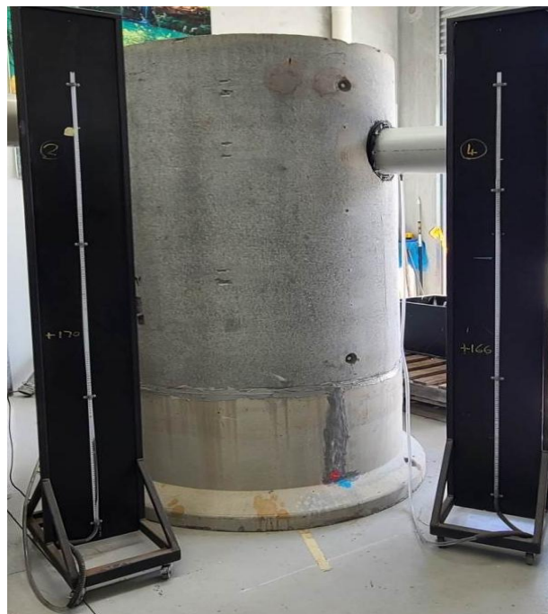
Figure 7 Manometers Installed at the Invert of the Inlet and Outlet Pipes to the HumeFilter
