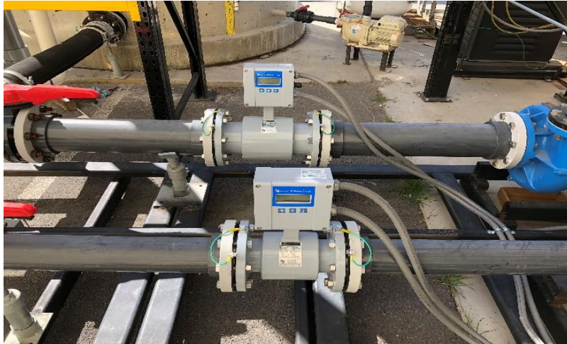
Figure 4 ModMag M2000 Electromagnetic Flow Meters
