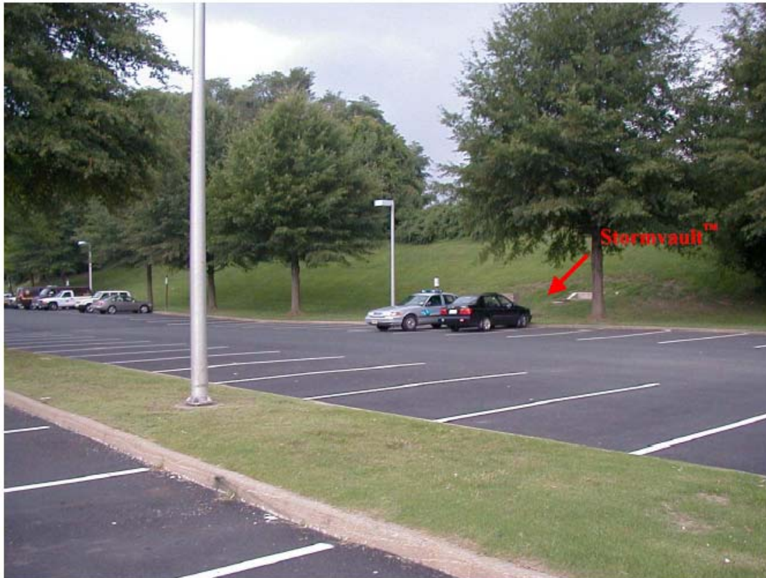
Figure 4. Site Drainage Area (from Yu and Fassman, 2001).
