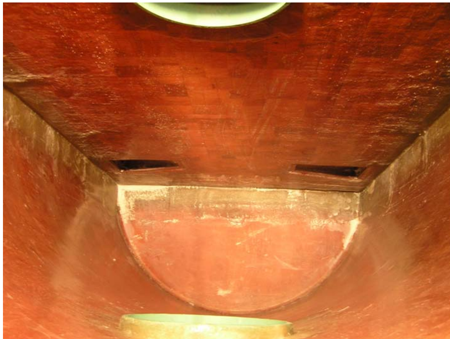
Figure 3 View of the baffle wall from the second compartment of the M2 manhole.
